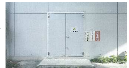
[宇品電気室防水扉(完成)]
